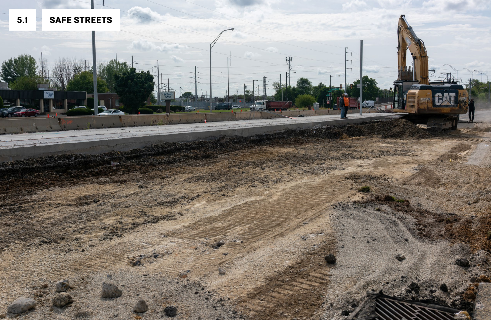
Shared trail construction on Island Avenue, September 2023.
