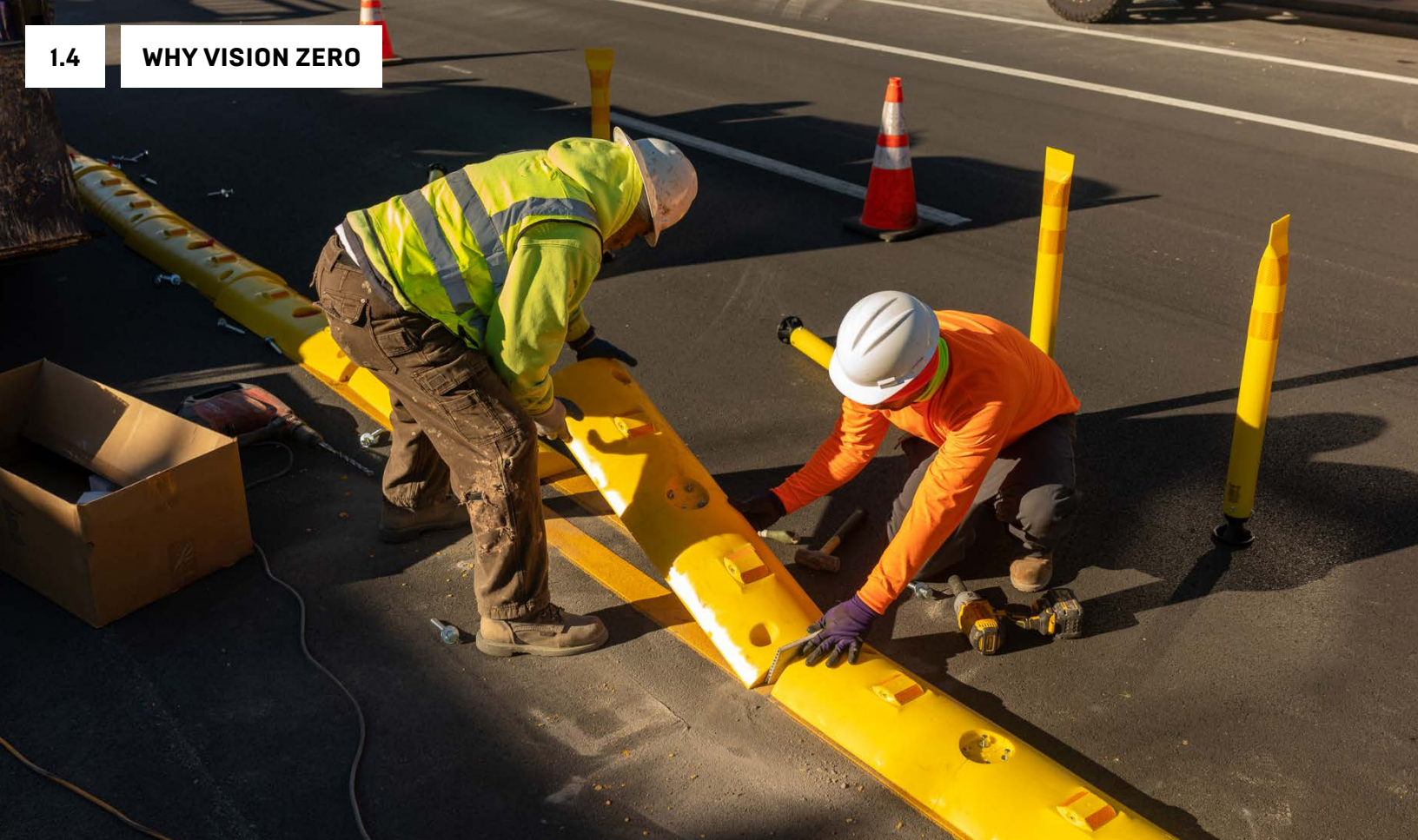
Hardened centerlines on Washington Avenue, November 2022
